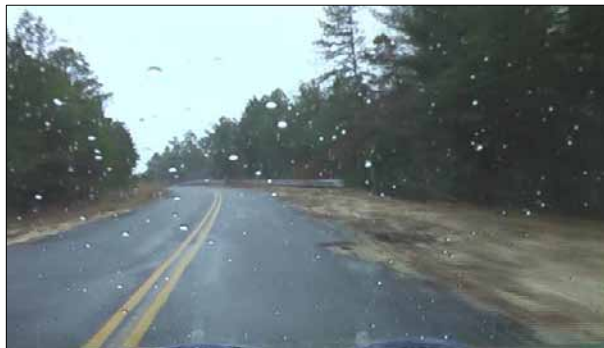
Photo 3. On this poorly maintained segment of Route 542, the edge has eroded.
