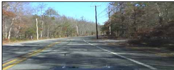
Photo 5. This utility pole on the inside radius clear zone poses a safety hazard on Route 610.
