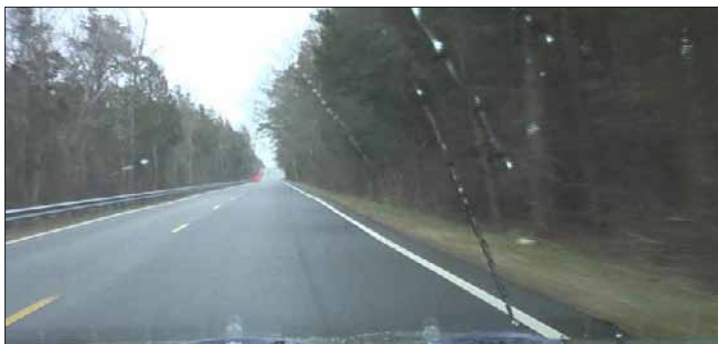
Photo 4. A narrow shoulder and clear zone poses a potential safety hazard on Route 623.
